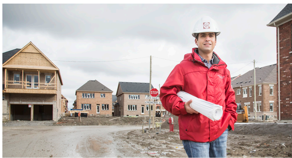
Boaz Feiner: Building a home can take 30 to 34 weeks from excavation to construction.
